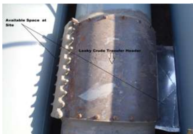
Figure I-3.2: Example of temporary safety measure to prevent new contamination from spill. The clamp is applied to stop a leak on a leaky pipe header running
