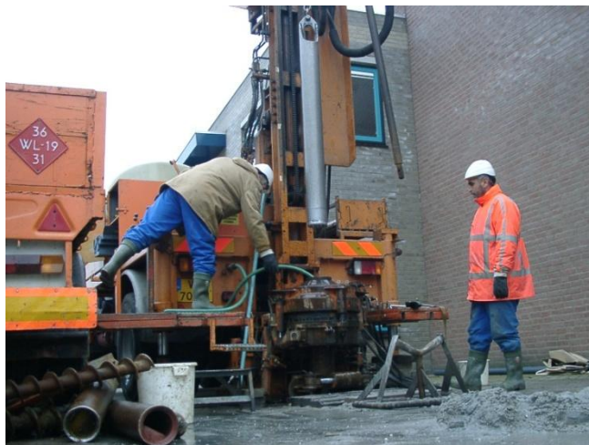
Figure III-2.2-ii. 13a, 13b and 13c: Examples of cased auger/pulse drill
