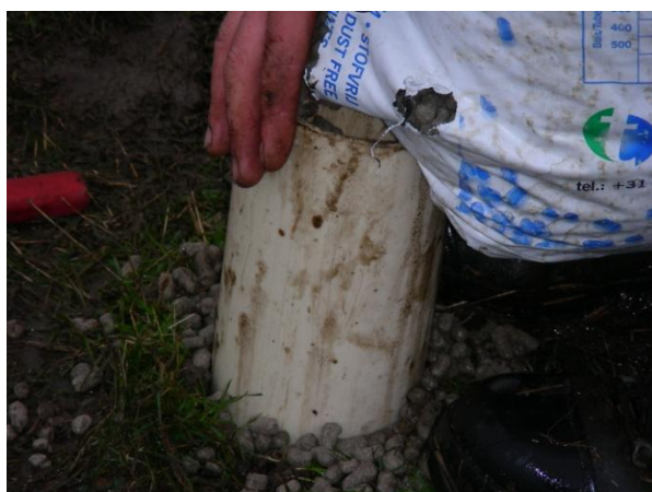
Figure III-2.2-ii.22a: Bentonite pellets
