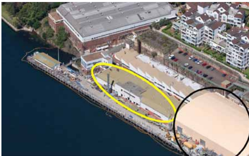
Picture 7. Remediation with odor control enclosure and treatment train. Source: Australian Federal Government (2013)
