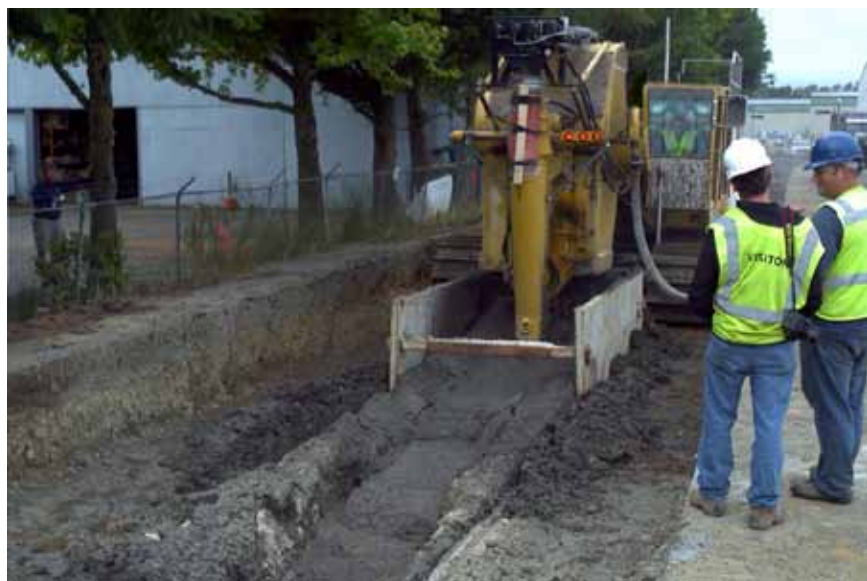
Picture 10. Combined trenching and slurry insertion.
